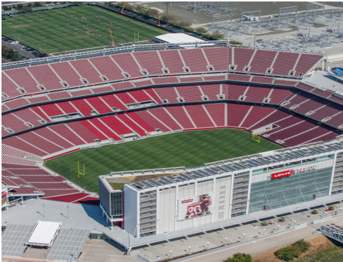
Levi Stadium. Photo courtesy of Clark Pacific.
